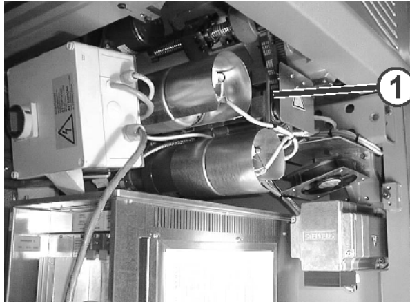
Fig. 2-26 Racking motor
